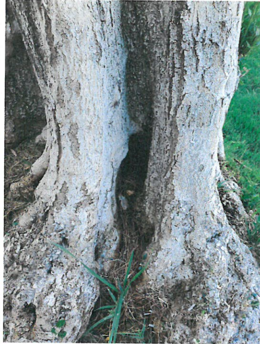
#73 (EO) Decay; continue to monitor
