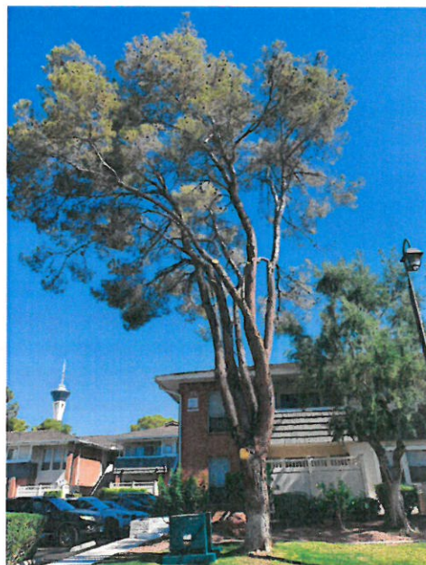
#N-03 (AP) Stressed, poor structure; remove and no replace due to utility box
